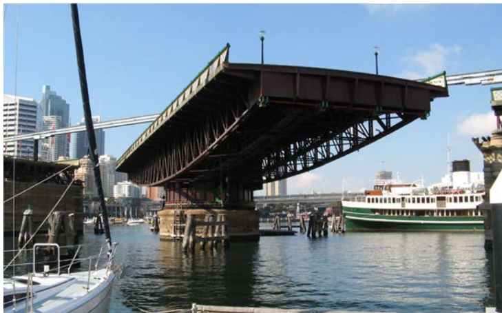
Pyrmont Bridge, Darling Harbour, Sydney was scheduled for demolition but lobbying achieved restoration, and its opening span is rotated every Sunday.
