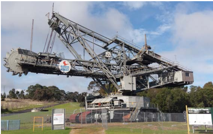
Bucket Dredger 21 extracted overburden and brown coal from the Morwell Open Cut 1955-92 in Victoria.
